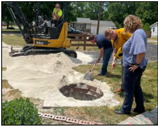
In 2023, a well is sealed in the Village of Wataga during the demonstration.
